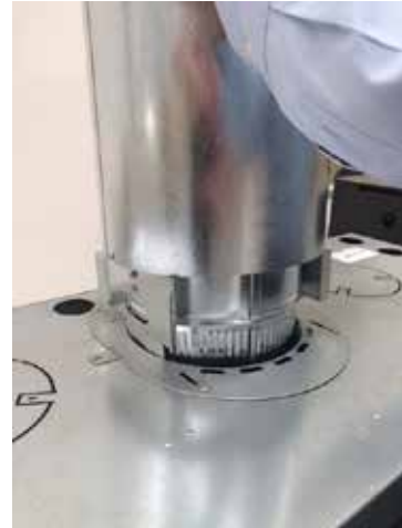
5. Air cooled bracket and pipe fitted to unit
